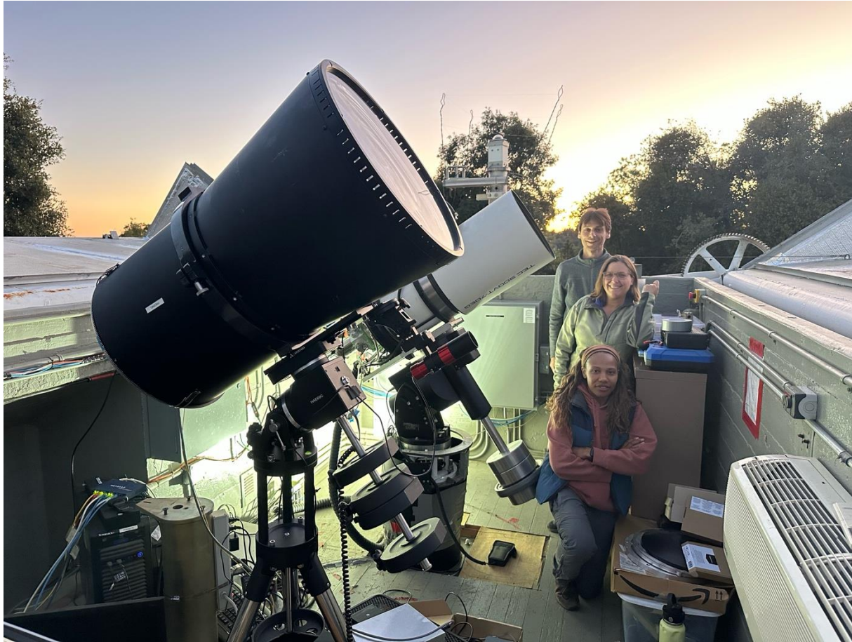
The first PANOSSETI telescope at Palomar, installed inside an existing dome.
